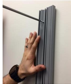
5. Using a level, make sure the height rod channel is plumb/straight. Mark the remaining four holes.
