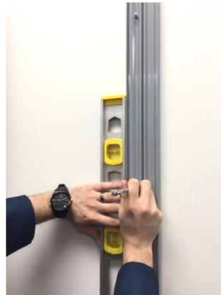
6. Swing the height rod channel to the side to drill lead holes into the marked locations. If mounting to drywall or plasterboard, obtain the four remaining drywall anchors and using a Phillips head screwdriver, insert the anchors into the wall.
