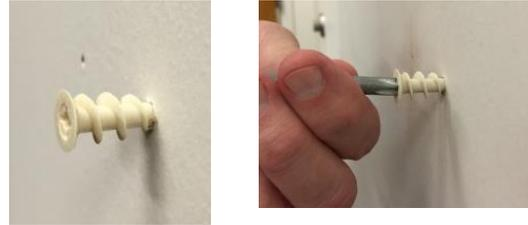
4. Obtain one of the 1 1/4" screws from the clear bag. Reposition the height rod channel against the wall, lining up the top hole with the inserted drywall anchor or drilled lead hole. Insert the screw through the front of the height rod channel into the drywall anchor or the drilled lead hole. Using a Phillips head screwdriver, tighten the screw until the height rod channel is held gently against the wall while still allowing it to swing freely from side to side.
